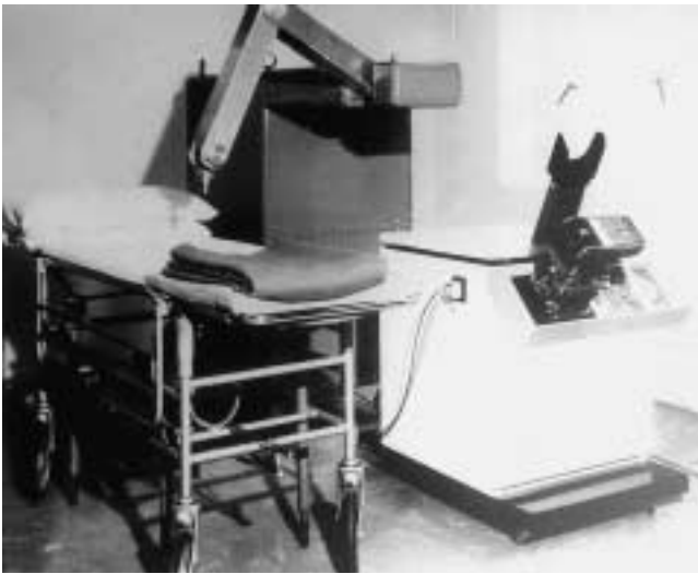
Figure 2 Scanner designed by Peter Wells, 1963–65, using electronics from the Disonograph
